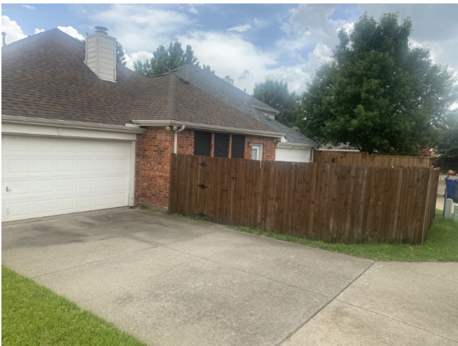
View from north rear of the home.
