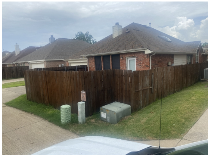
View of the south rear of the home.
