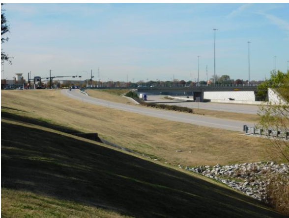
Looking towards SH 190 from east of the site, the subject site is to the left on this photo
