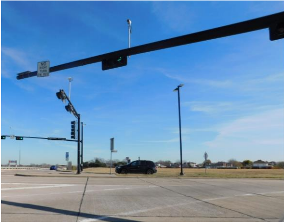
Looking to the site at Firewheel Parkway and SH190
