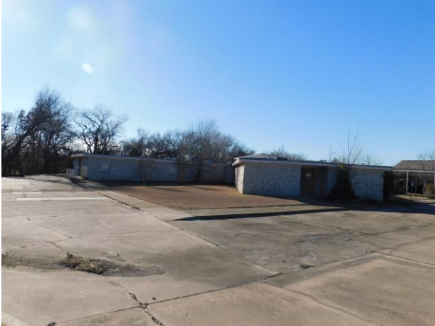
View of subject site from Castle Drive
