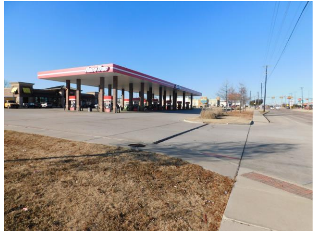
View north at adjacent RaceTrac Gas Station
