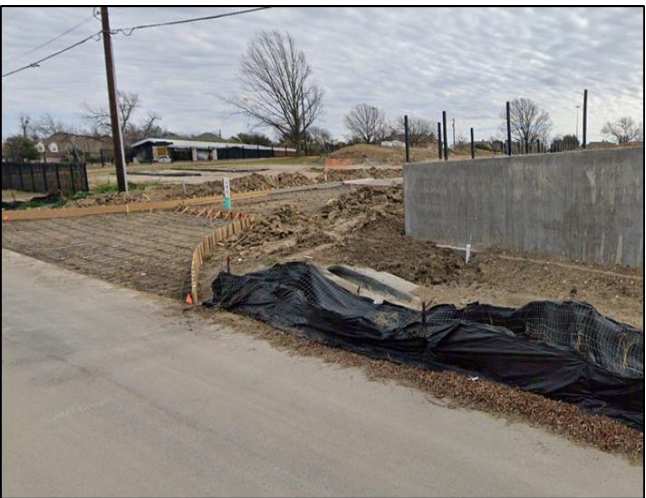
View of the site currently under construction.
