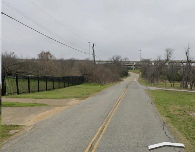
View of Zion Road Frontages looking west towards the subject site on the left beyond the fence.
