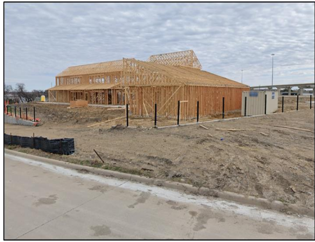
View of the site clubhouse under construction.
