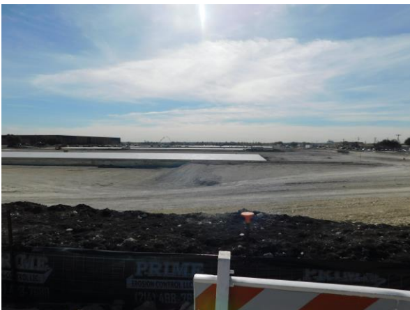
Industrial development under construction to west of the site
