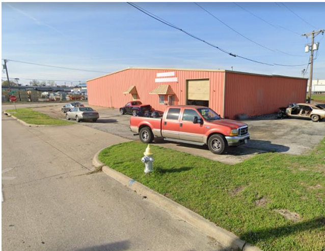
South of subject property from Lonnecker Drive.
