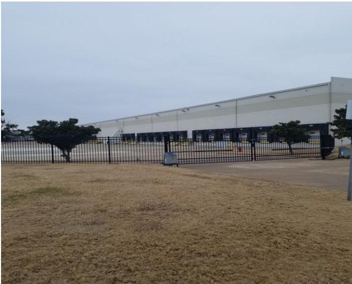
Looking at the rear elevation of the building (truck court).
