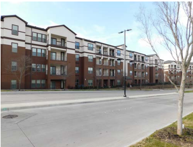
View of The Mansions at Spring Creek from the subject property
