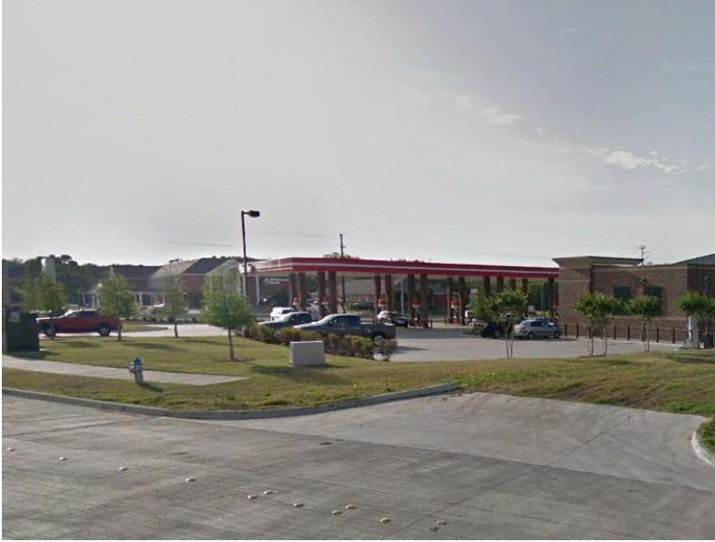
Looking east at adjacent property across Guthrie Road from subject site.
