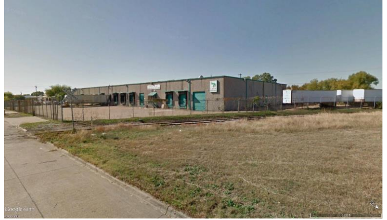
Looking southwest at the north and eastern portion of the subject site from Miller Park Drive.
