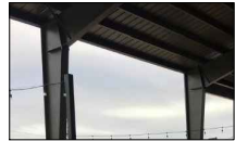
PRE-ENGINEERED METAL STRUCTURE
