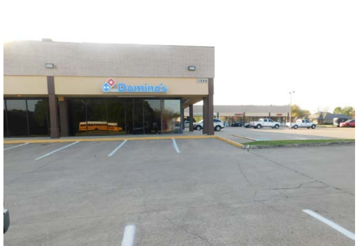
View of properties located on the east corner of Hayman Drive and Rowlett Road.
