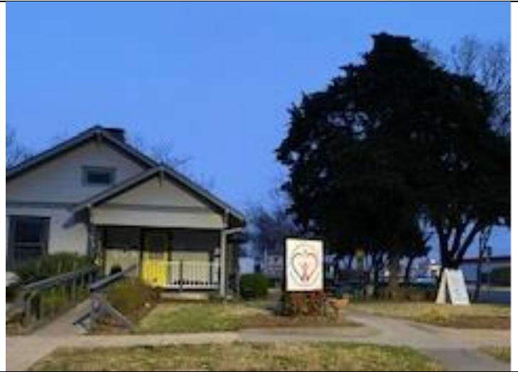
Looking at subject property from Twelfth Street
