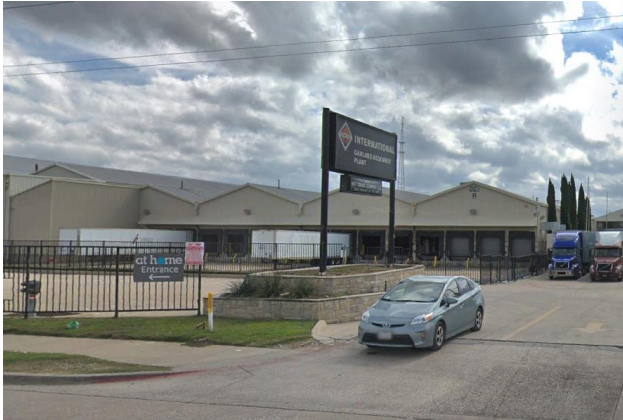
View of site looking west on Forest Lane
