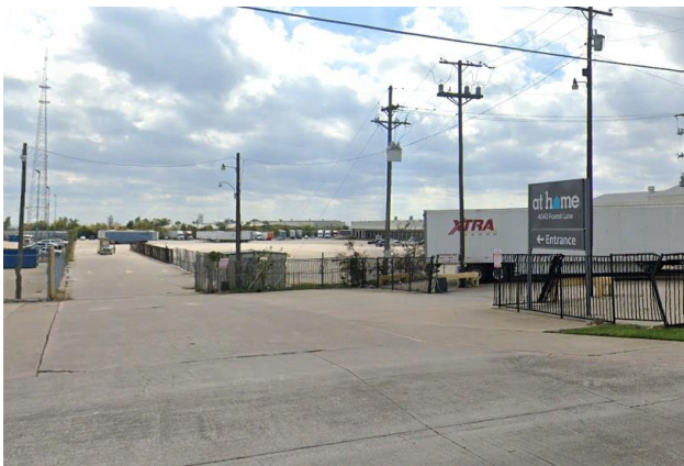
View of site at east entrance on Forest Lane
