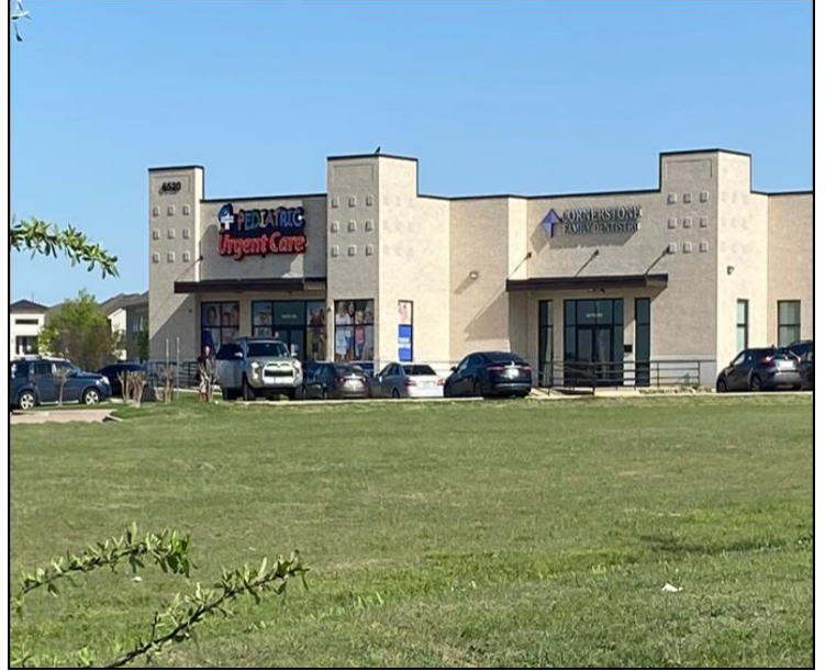
West of the subject property along North President George Bush Turnpike.
