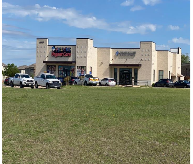
West of the subject property along North President George Bush Turnpike.
