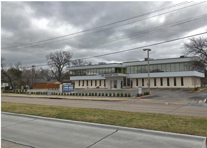
View of office property located to the north, across Broadway Boulevard.
