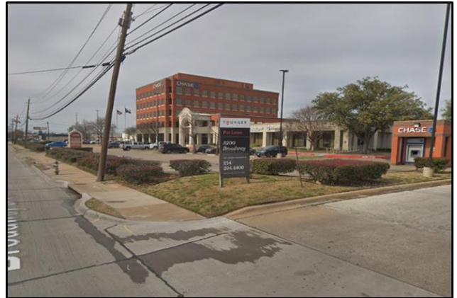
View of the property from the east.
