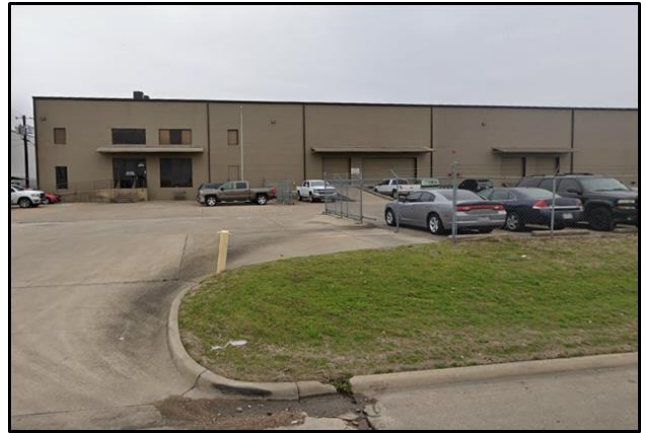
View of the property northeast of the site on Sherwin.
