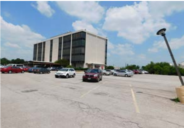
Looking north from subject property
