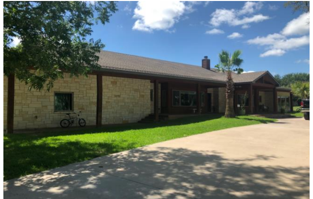
Looking at the existing house on proposed Lot 1.
