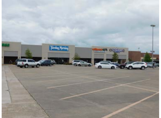
View of existing shopping center on the subject property.
