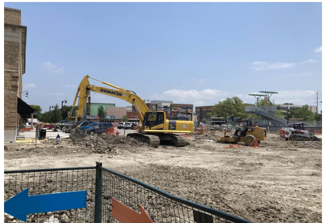
East of subject property (Downtown Square construction)
