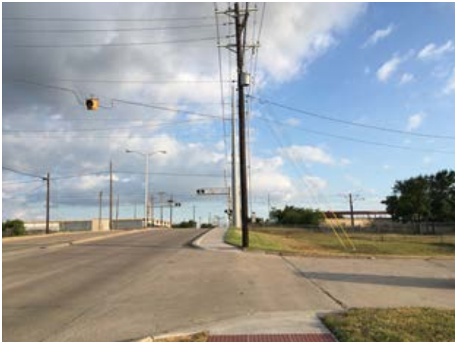
View of the DART rail from Shiloh Rd. and subject property.
