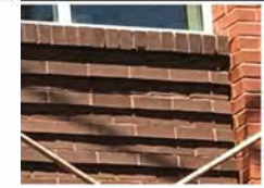
Staggered Brick Detail
