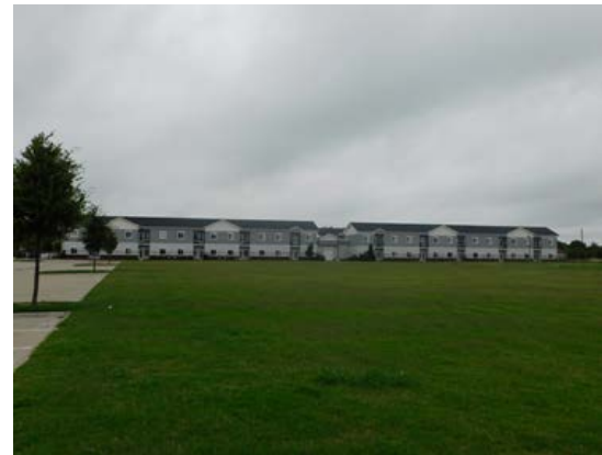
Looking the existing charter school dormitory
