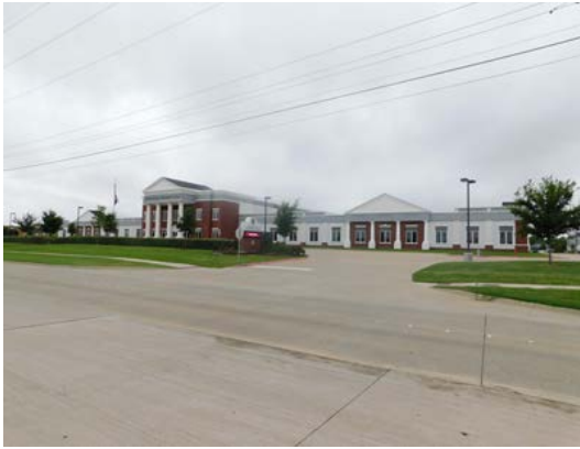
Looking at the existing school building
