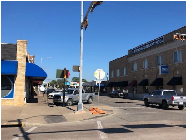
Looking west of the subject property
