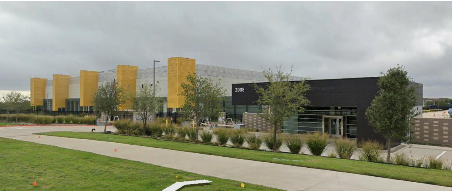
Data Center (Employment) along Lookout, west of Campbell Road
