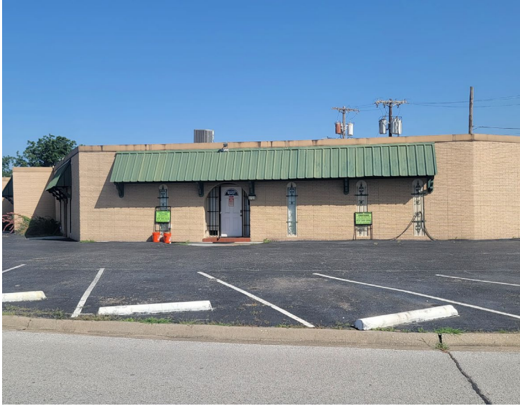
View of the subject site looking North.
