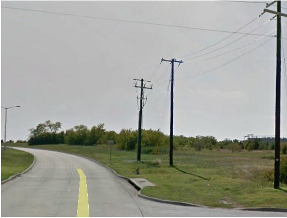
Transition Zone at the southwest corner of Campbell Road and Lookout Road
