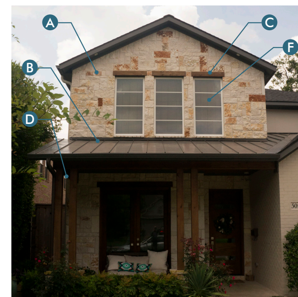
A Local stone cladding; B Standing seam metal roof; C Heavy timber or monolithic stone lintels; D Simple square porch posts; E Post brackets; F Modern horizontal window panes; G Traditional vertical window panes
