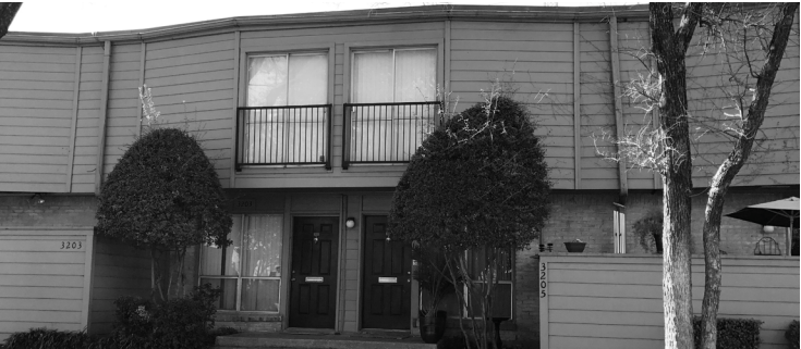
Balcony has no base making it unusable and inappropriate.
