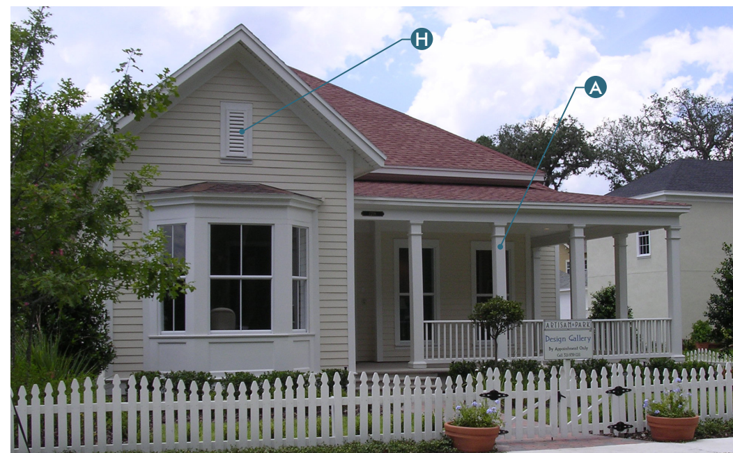
A Prominent front porch; B Bracket detail on rake; C Exposed rafter tails; D Eave returns; E Gable pediment detail; F Shed dormer; G Stone accent on chimney; H Gable vents or windows
