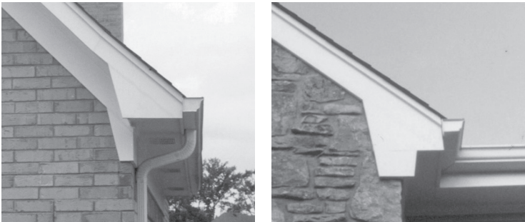
Deep overhangs should not terminate with an oversized "box" cornice detail or large cornice return.
