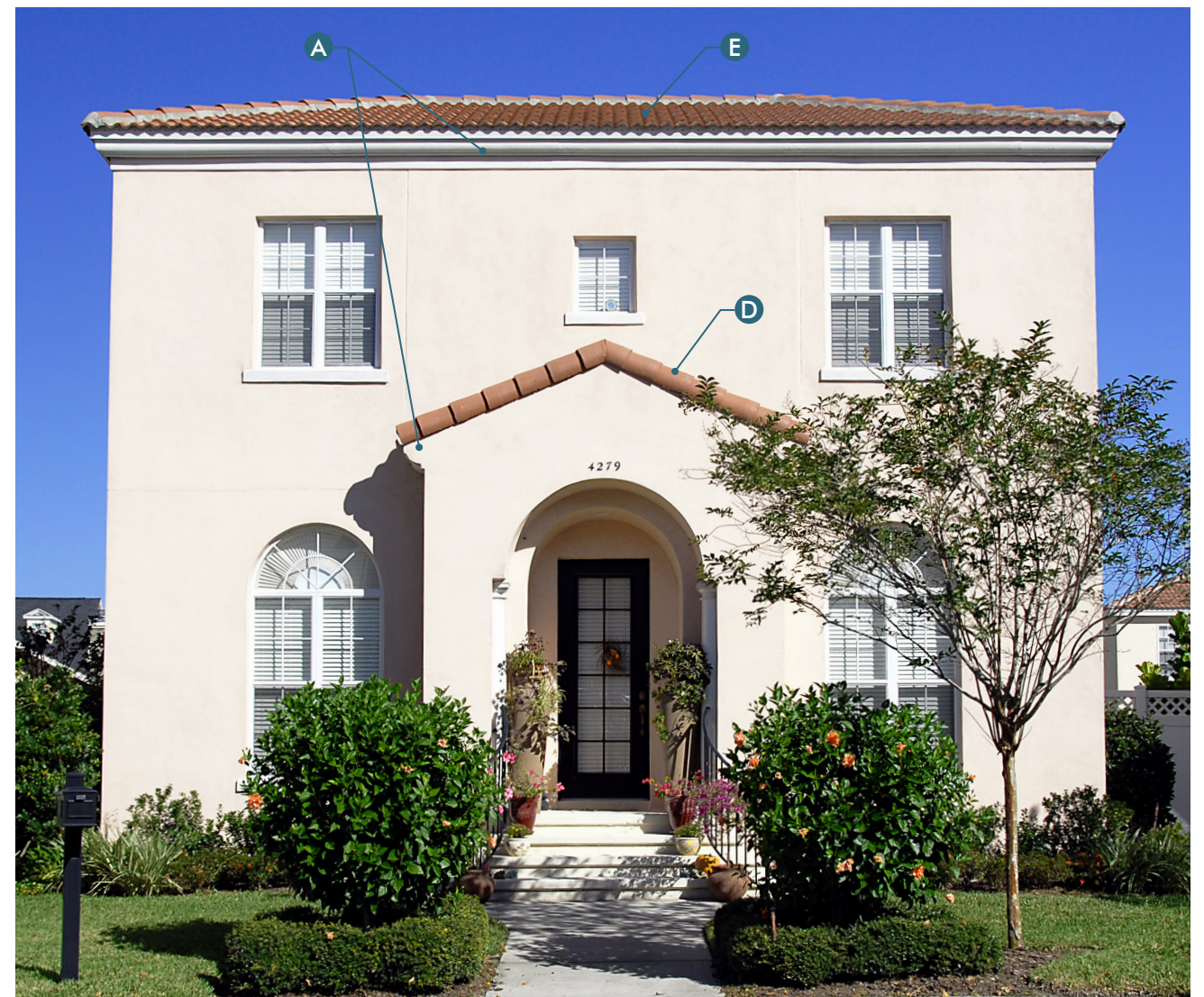
A Shallow eave with stucco profile; B Exposed rafter tails; C Eave brackets; D Rake tile detail; E Barrel tile roof; F Barrel tile gable detail; G Board and batten shutters
