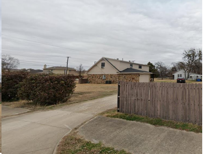
Looking at the subject property from South Country Club Road
