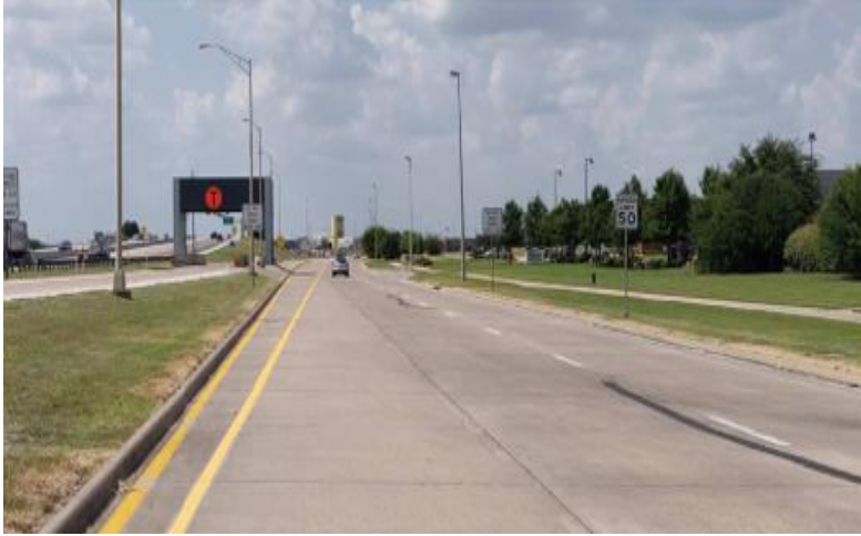
View from South East Service Road
