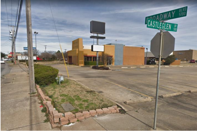
View from the corner of Castleglen and Broadway of existing structure.
