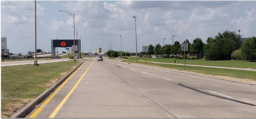
1 VIEW FROM SOUTH EAST SERVICE ROAD
