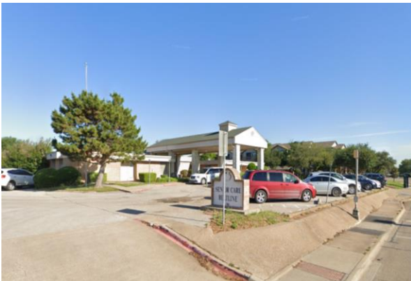
South of the subject property.
