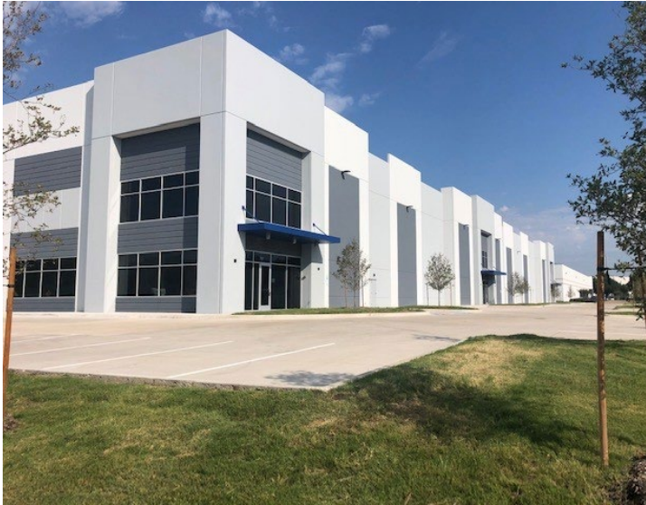
View of the subject site, looking north.
