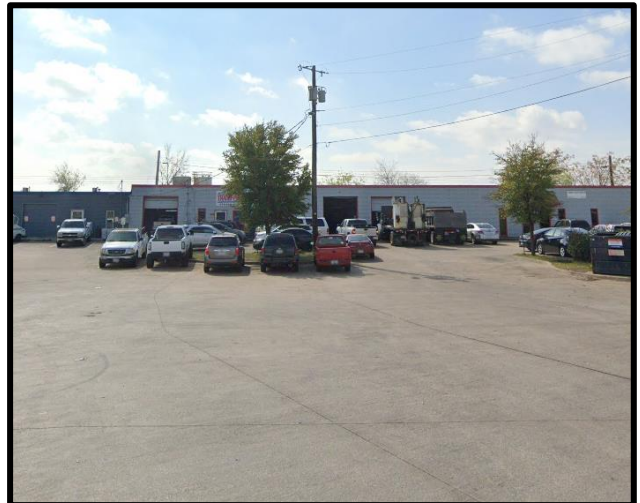
South of the subject property.
