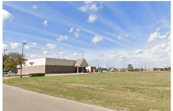
West of subject property from Crist Rd.
