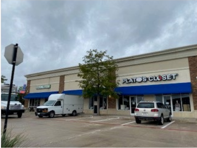
View of the subject property from Horton Way
