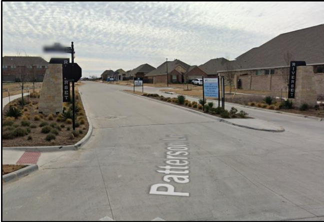
View of the subject property from Buckingham Road.
