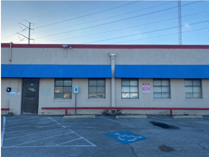
View of the subject site West from North First Street
