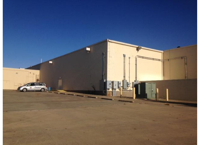
View of rear of subject site building.
