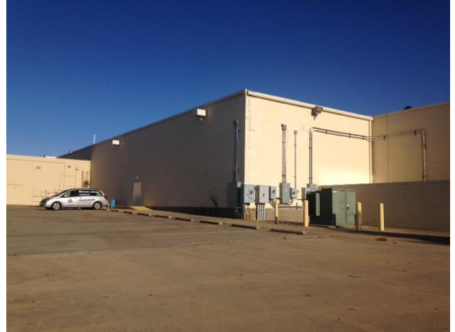
View of rear of subject site building.
