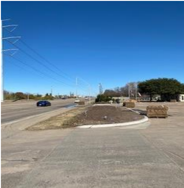
Looking north along site and Lavon Drive.
