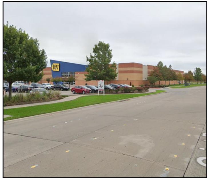
Looking east of the subject property from Crist Road.
