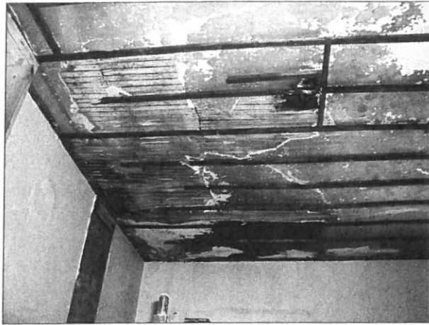
Fig. 7-11. Lath and plaster can offer more resistance to fire than modern drywall.
