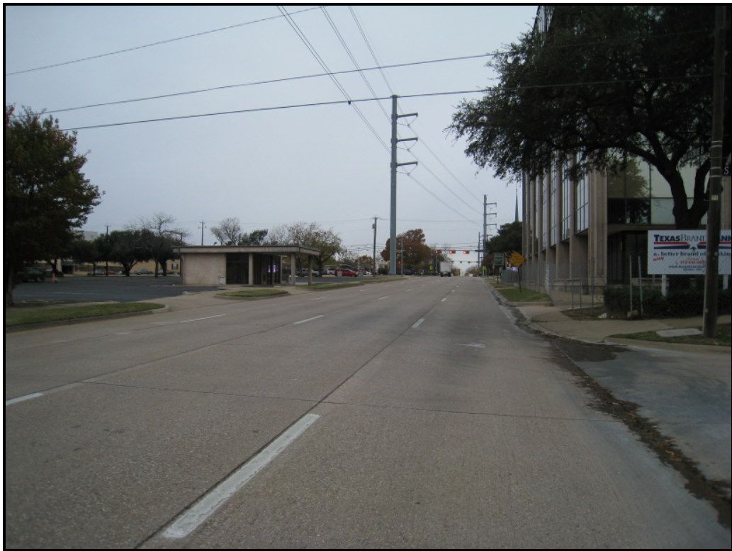
Viewing west along W Avenue B from 7th Street
