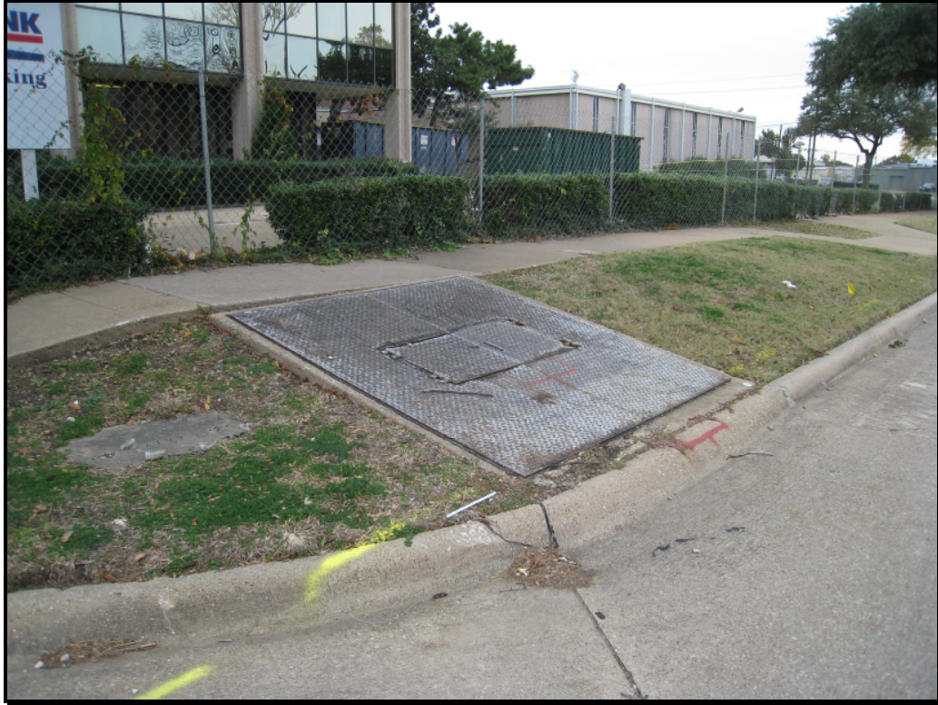
On-site utilities at northwest corner of W Avenue B and 7th Street
