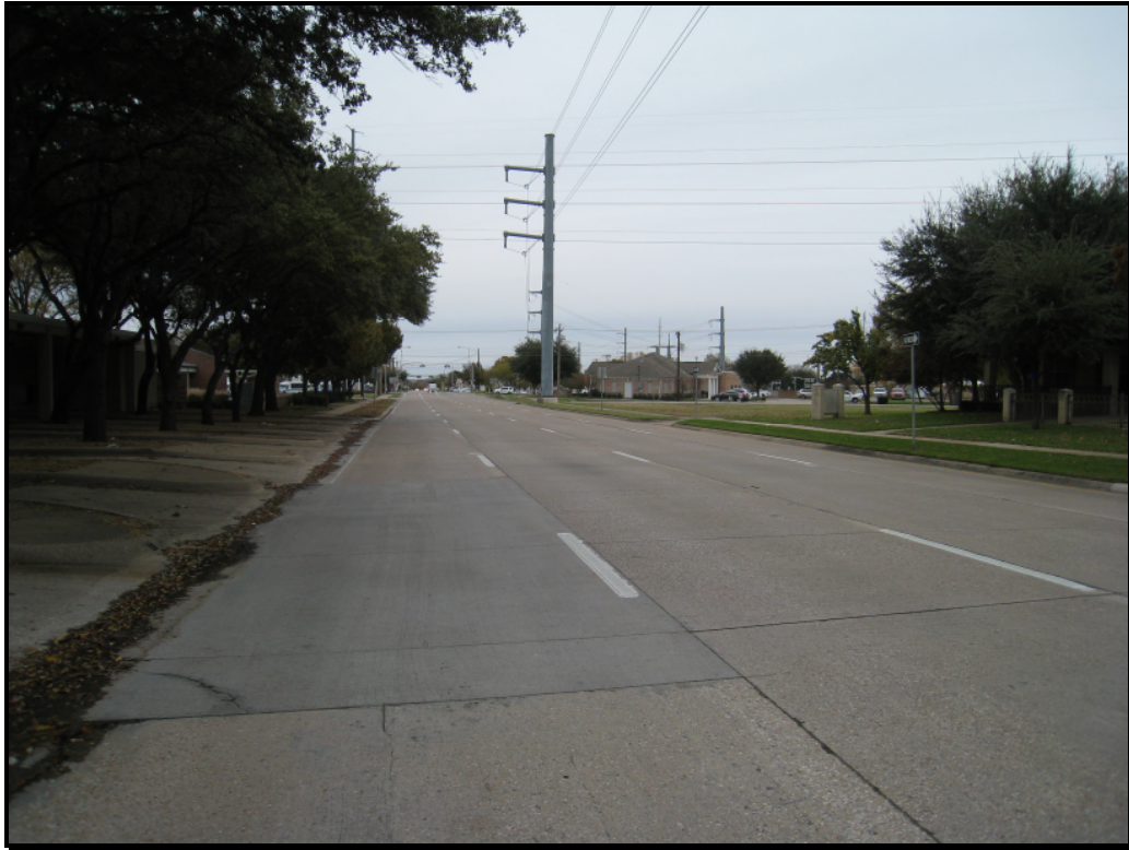
Viewing east along W Avenue B from 7th Street
