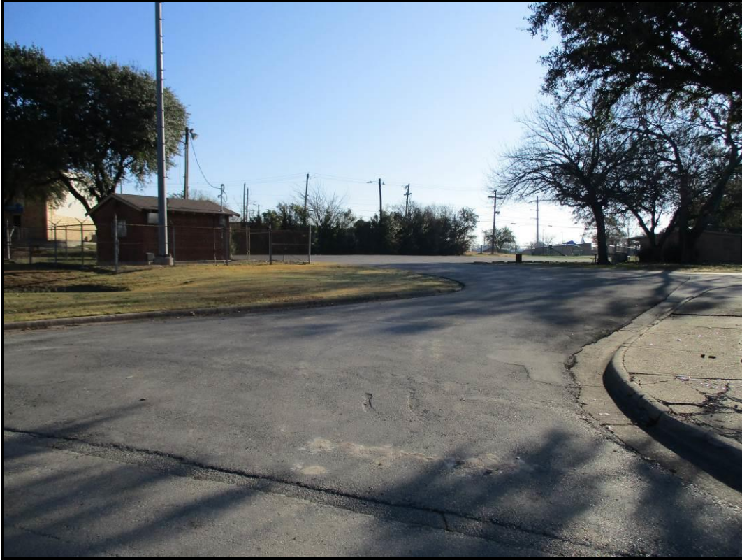
Looking northeast at proposed permanent utility easement 1.
