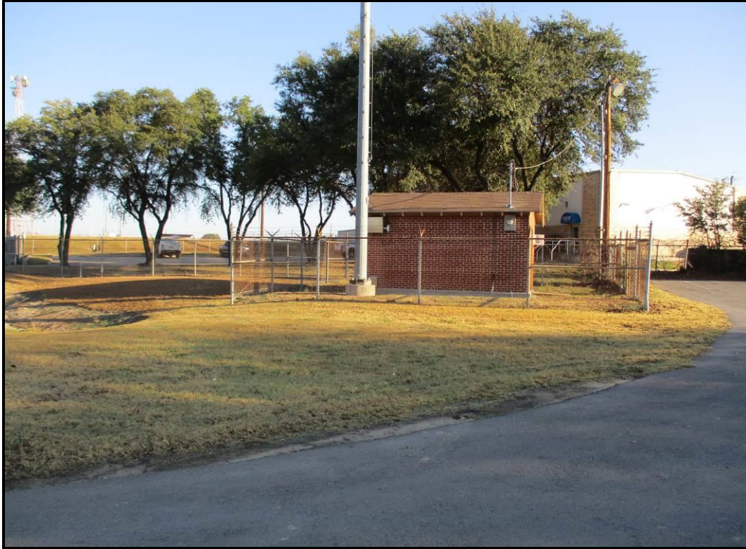
Looking northeast at proposed permanent utility easement 2 (existing station inside fence).
