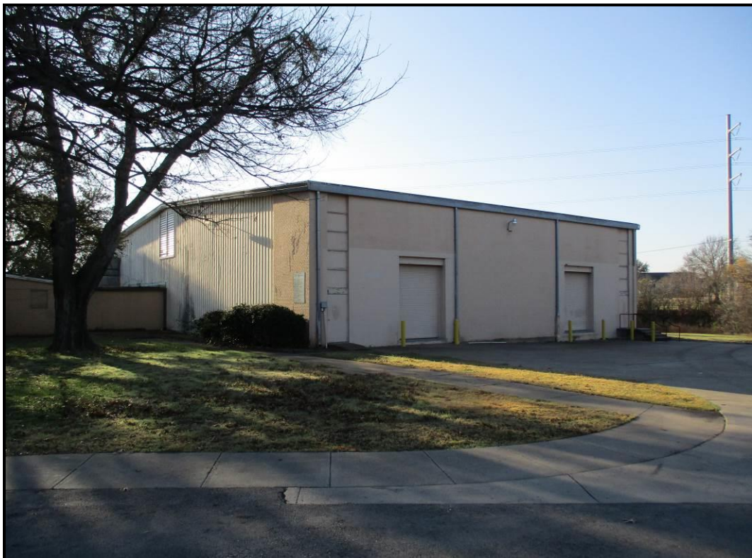
Looking southeasterly at subject building from proposed permanent utility easement 1.
