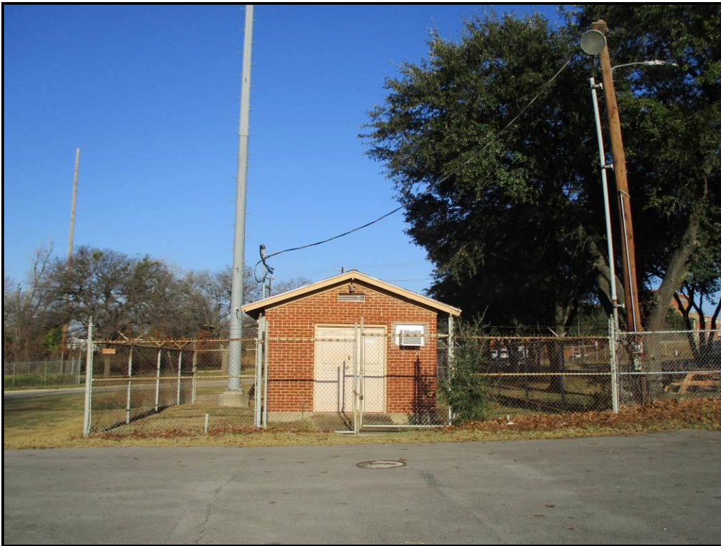
Looking northwesterly at proposed permanent utility easement 2.
