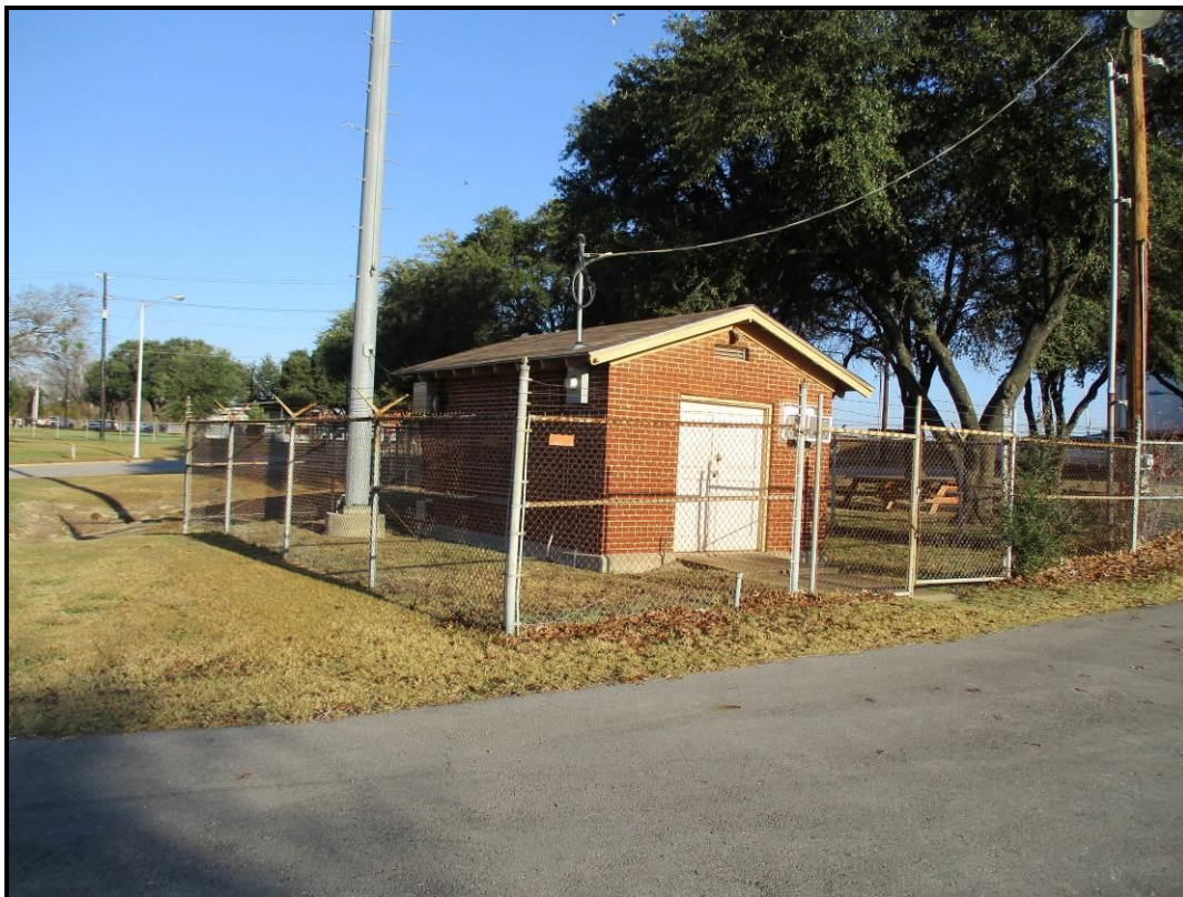
Looking northwesterly at proposed permanent utility easement 2.
