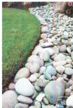
Install 5"- 6" River Rock to cover bare areas and provide a consistent aesthetic and reduce erosion.
