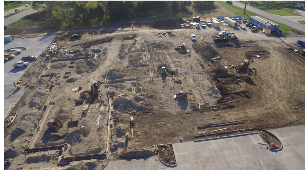
Animal Shelter under construction
