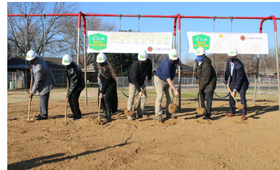
Playground Replacement Program Groundbreaking
