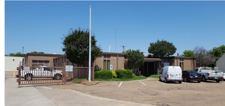
Transportation Maintenance and Operations Facility
