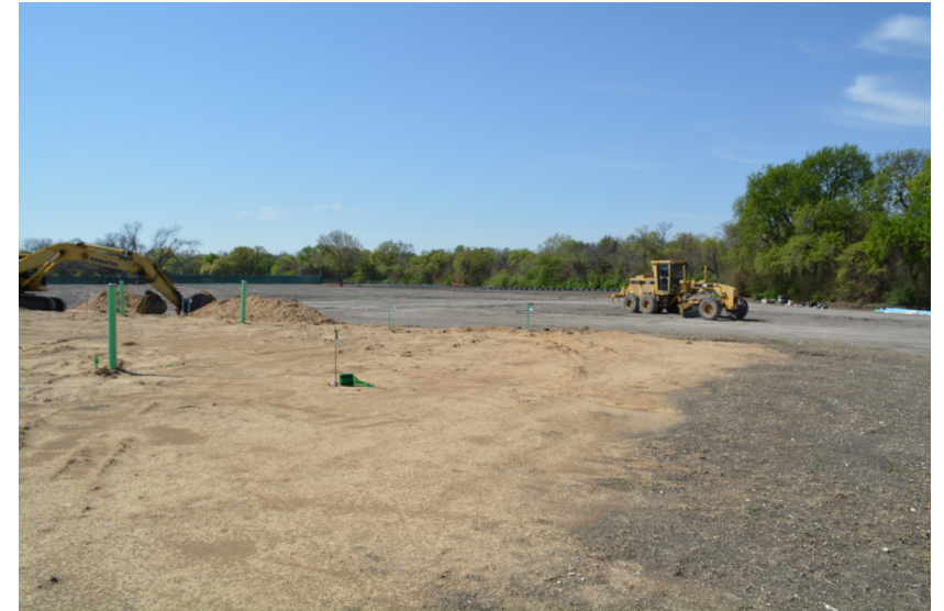
Rick Oden Park under construction
