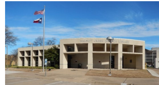
Existing Walnut Creek Branch Library
