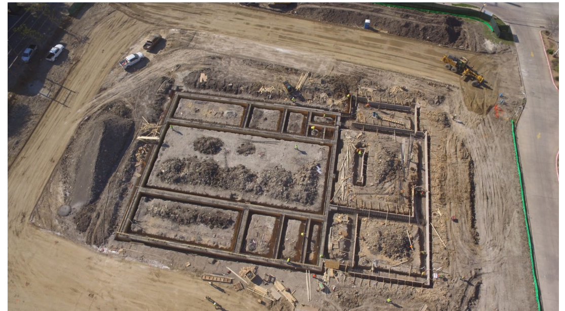
Police Property and Evidence Building under construction
