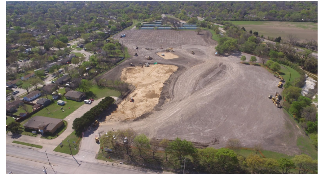
Rick Oden Park under construction
