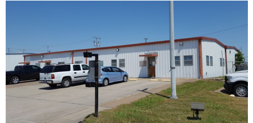
Street Department Facility
