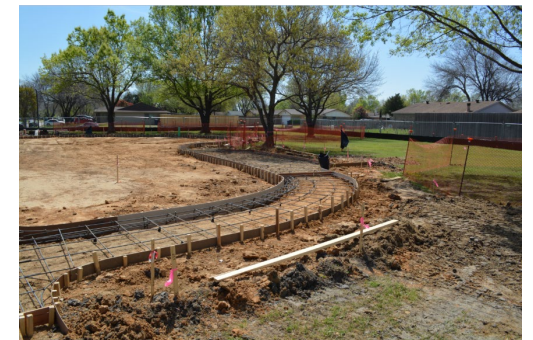
Bob Hall Park under construction
