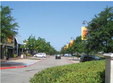
Roadway and Site Improvements
