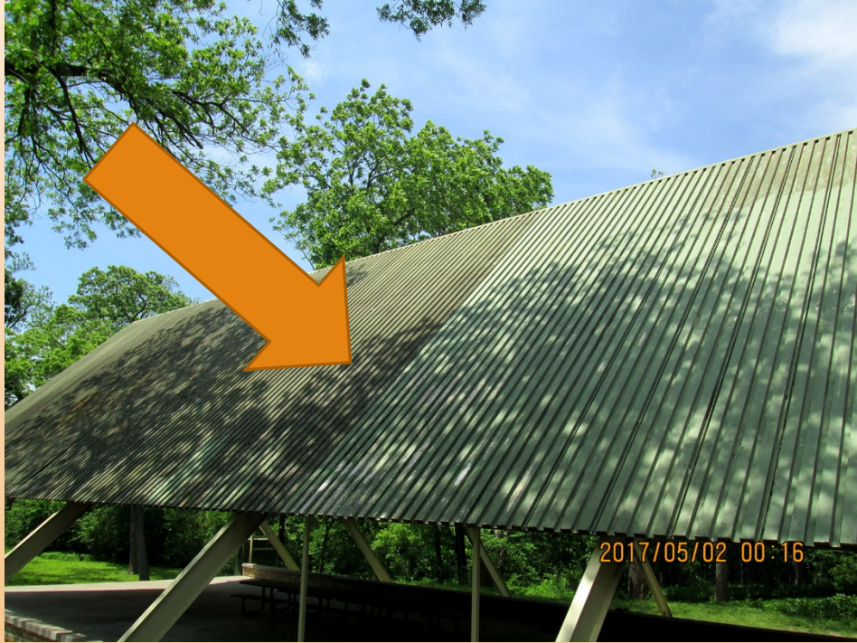
Paint It Up – Pavilion Roof Before and During Power-washing
