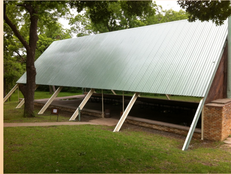
AFTER – Roof Repainted
