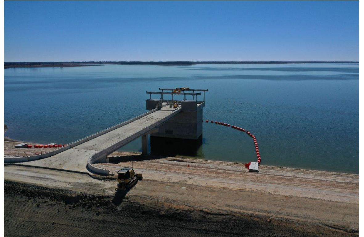
Intake Tower Construction and Wet Side Impoundment
