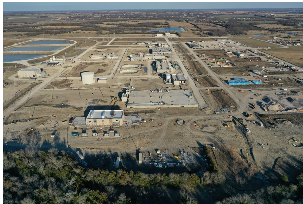
Leonard Water Treatment Plant
