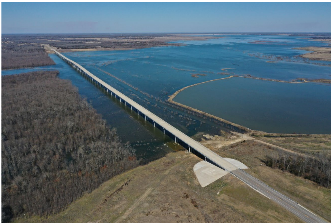
FM 897 Bridge Complete and Open
