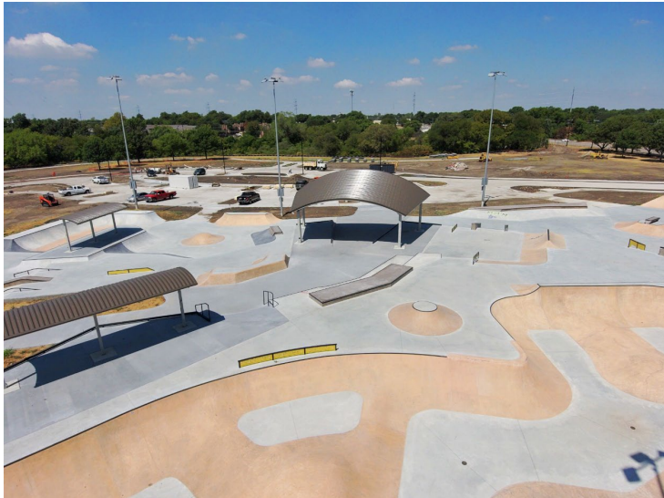
Rick Oden Park skate park construction progress August 2022
