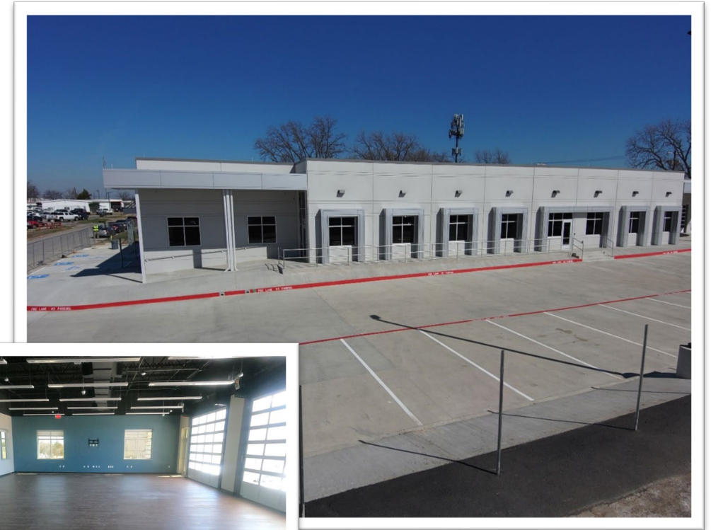
Construction progress photo of new facility
