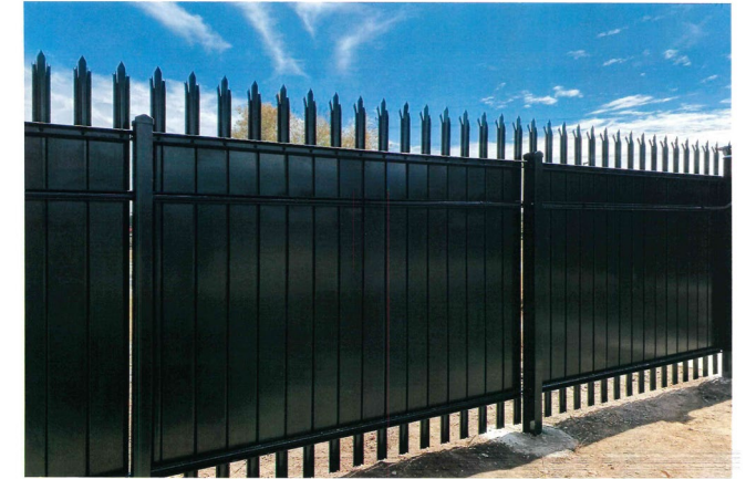
Perimeter Fence – construction progress photo
