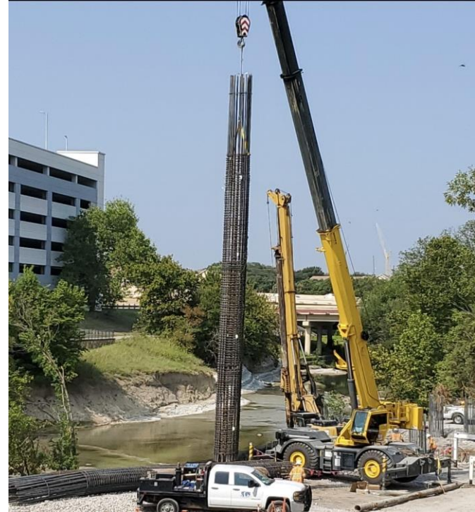
US 75 Bridge: Setting Cage for Bridge Pier
