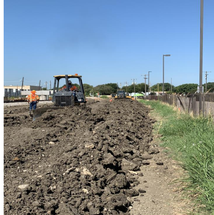
Grading for Shoo-Fly Rail Josey Bridge Location
