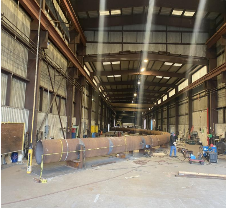
Midway Bridge Arch King Fabrication - Houston, TX
