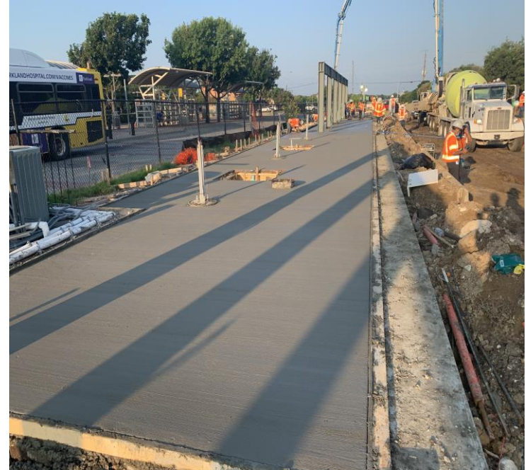
Addison Station-North Platform Completing Concrete Placement
