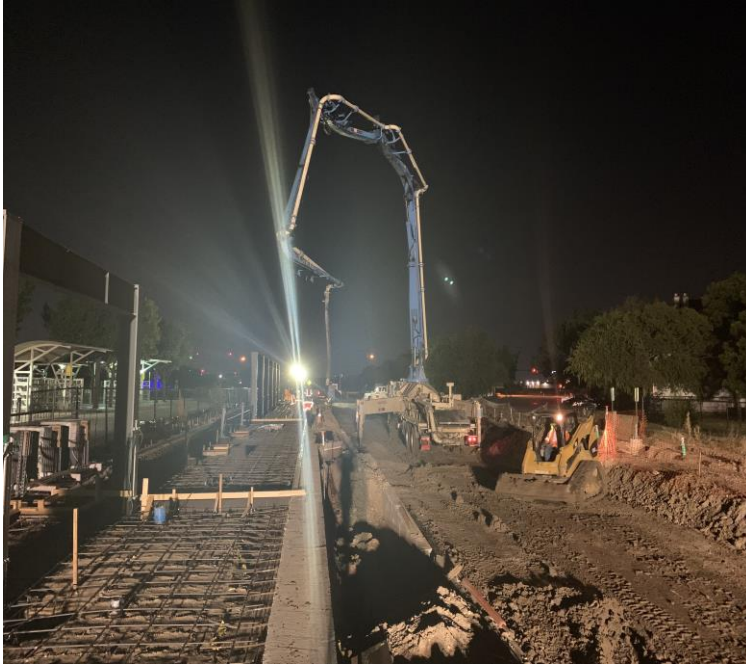
Addison Station-North Platform 4:30 a.m. Concrete Placement
